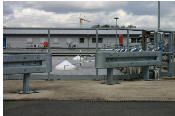
Figure 4: Collection Hoods at Erlangen WWTP
