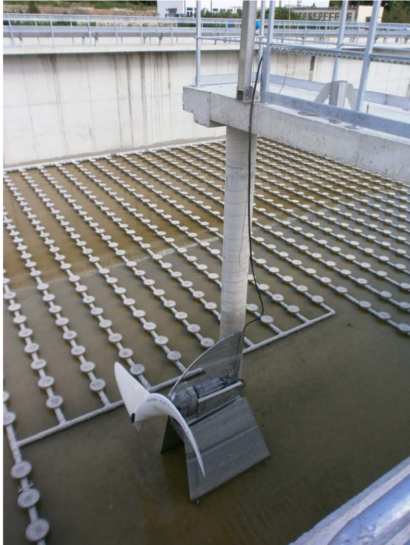
Figure 3: Top view - CYBERFLOW ® - Accelerator & iDISC ® - Membrane Aerators during installation
